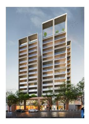
The façade treatment is robust and integrated into the structure and form of the building which results in a façade that present as strong and well proportioned. Strong vertical concrete elements work in conjunction with the horizontal repetition of the balconies. Light weight 'add on' elements have been avoided and façade details have been created from precast concrete elements that provide shadow details and shifting scales and rhythms that add visual interest.
